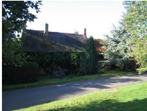
Poplars Farm is a large historic building but sits low in the ground south of The Green
