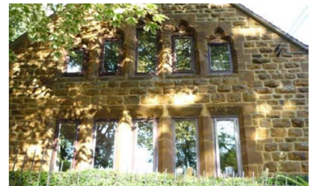
Gothic revival windows at The Old School partially surviving conversion
