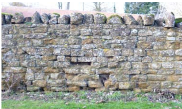
Typical ironstone boundary wall
