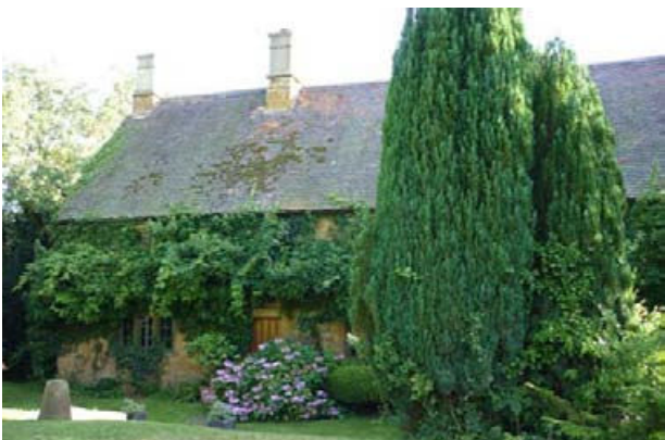
Poplars Farm house is partially obscured by greenery
