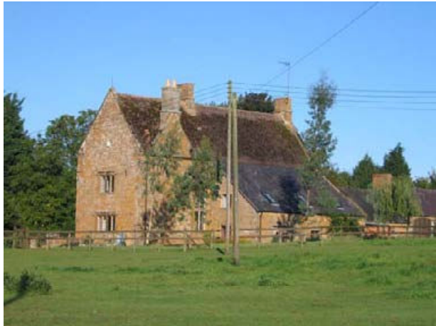
The later extension at Mansion House Farm has a Welsh slate roof
