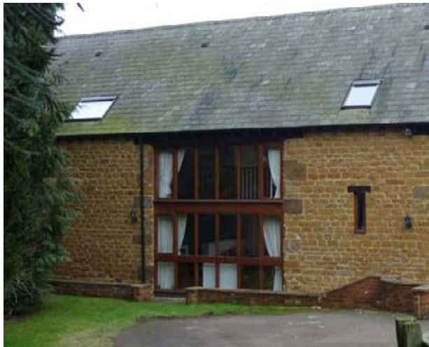
Former barn door opening retained
