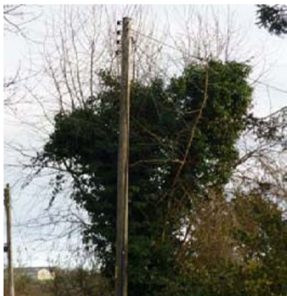
Tree interfering with overhead lines
