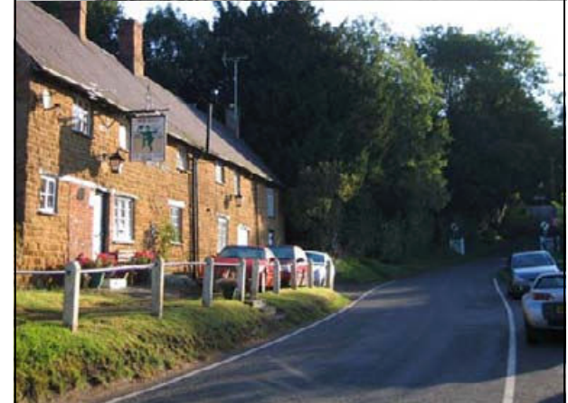
The Green Man PH has lost its thatched roof and a building on the south side of Holloway was demolished in the mid 20th century, presumably to widen the highway, but otherwise little has changed. The upstairs of the building has served as both the Oxfordshire Courthouse for the Inclosures Act and as the village hall meeting room.
