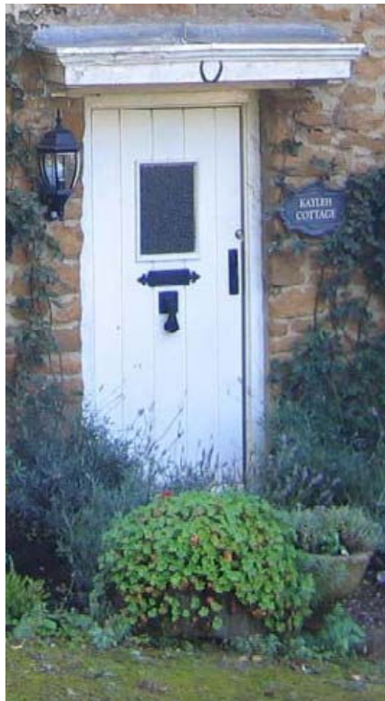
Traditional plain plank door with timber plain canopy
