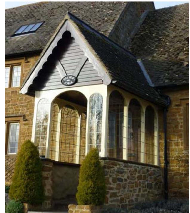
Prominent porch at The Forge
