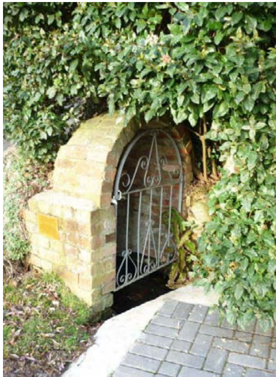
Wells, cisterns and pumps are an important feature of the village
