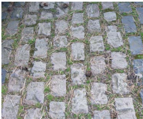
Small areas of granite blocks exist
