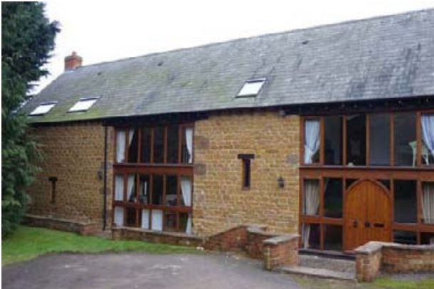
Mansion House Barn
