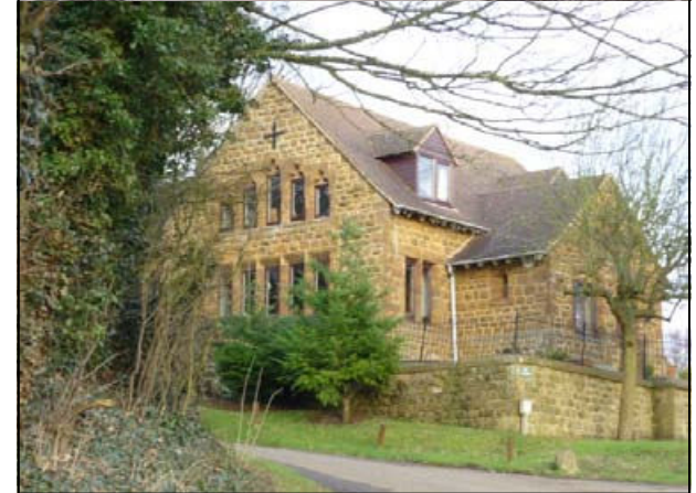
The conversion of the former Church of England National School into a dwelling has entailed splitting the fine trefoil gable windows and the insertion of a dormer window to accommodate an upper floor. The railings have been retained and the former use is still discernable, although the loss of the school bell is regrettable.
