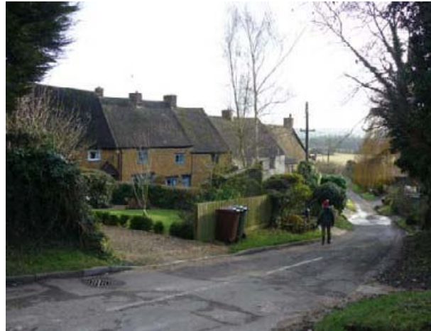
2 This terrace of cottages is not listed but are the best surviving example of 18th century labourers' cottages. Two storeys and constructed from coursed ironstone rubble they demonstrate the use of local building material in the construction of the most humble type of dwelling. The loss of original casements, the rendering of one cottage and car parking detract from this frontage which forms an important corner of the village green.
